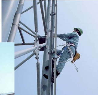
FM Skylock installed on the transmission tower
